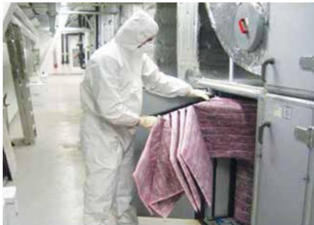
Figure 9: Personal protection equipment for filter replacement
